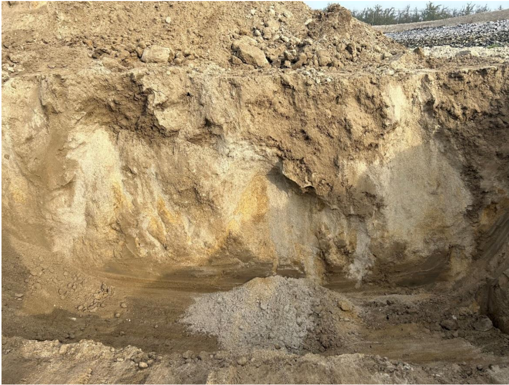
Figure 6 RIB 2 Test Pit Permeability Testing Location December 2023
