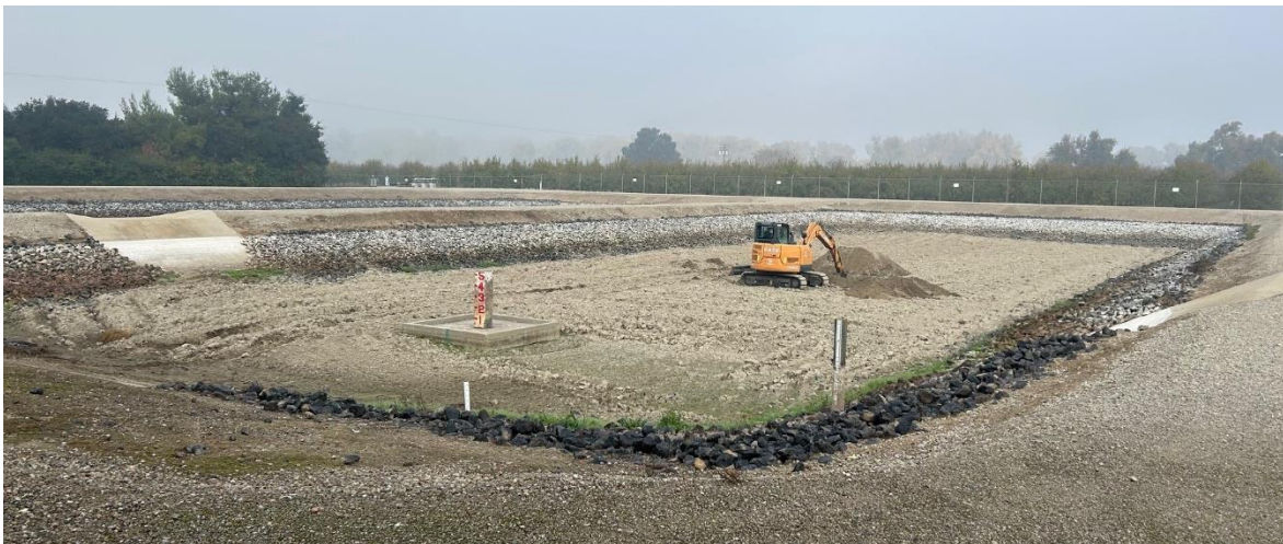
Figure 5 RIB 2 Test Pit Location December 2023
